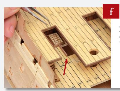
Cut a 20mm length of 2 x 2mm wooden strip. Glue it into place as shown, running from the grating and along the edge of the hatch.
