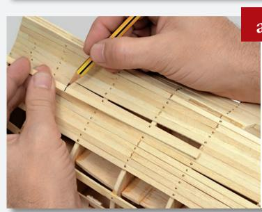
To fill a gap between planks in the hull, take a 2 x 5mm plank
